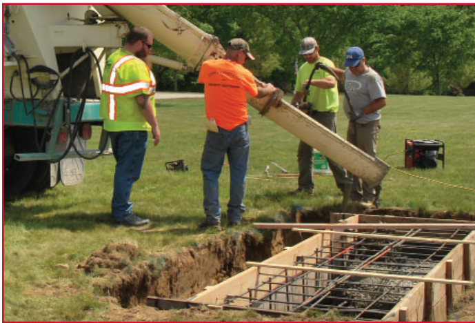
On June 2 nd , a crew excavates, then pours the base, for the Rhode Island Gold Star Families Memorial Monument at the Veterans Cemetery in Exeter.
