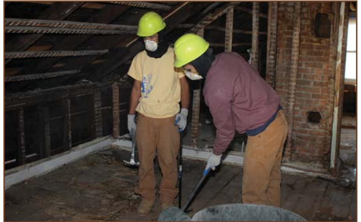
Students work to remove five layers of flooring to get back to the original hardwood..
